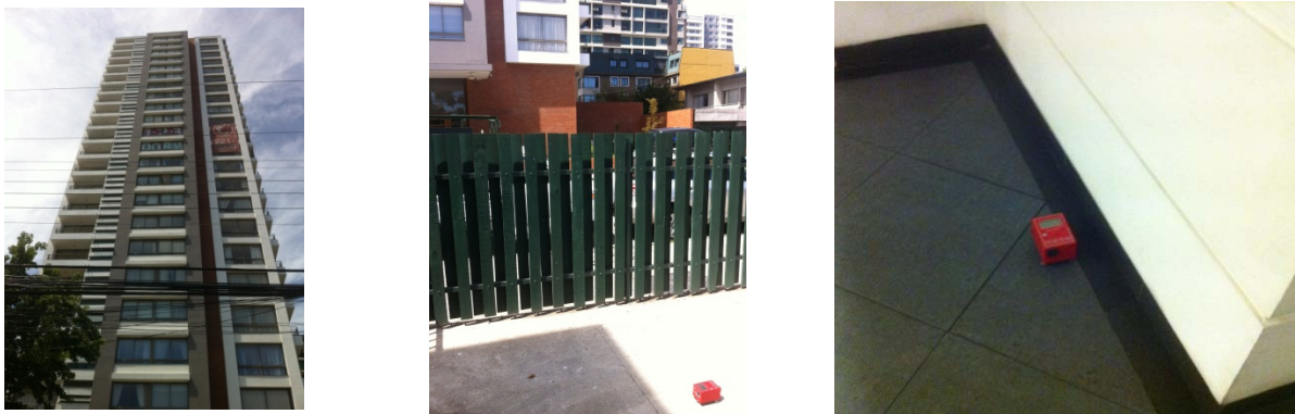
Fig. 5 – Elevation of 24 Storey Building and ambient vibration measurements
