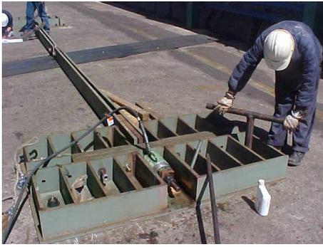
Fig 9 Final tighten of nuts to the floor slab
